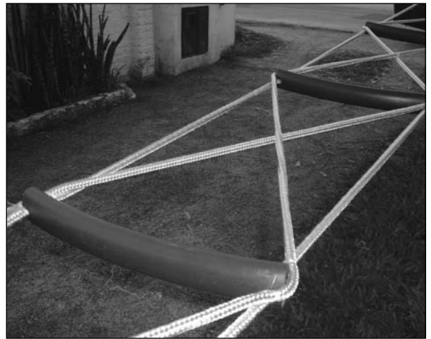
Figure 4. String bridge, 'ship ladder' model, before being installed in Lami, Porto Alegre. (Photo by L. X. Lokschin).
